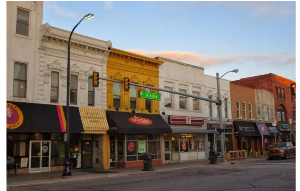
Figure 136 | Rehabilitated storefronts showcase visible stabilization, quickly increasing resident confidence | Unnamed photographer
