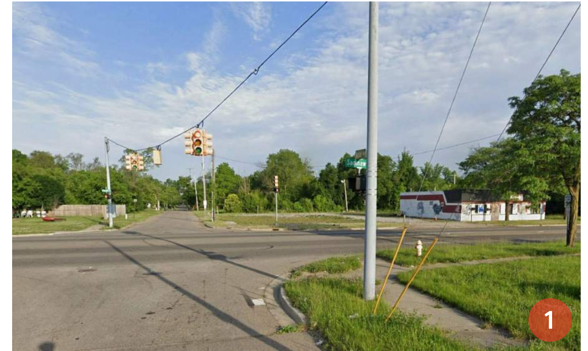
Figure 28 | Major intersection with limited visible crosswalk markings and minimal pedestrian-focused design elements | Google Earth 2025
