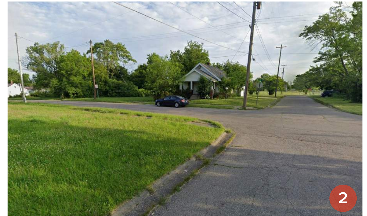
Figure 26 | Cracked and discontinuous sidewalk within a residential street, illustrating gaps in neighborhood-level pedestrian connectivity | Google Earth 2025
