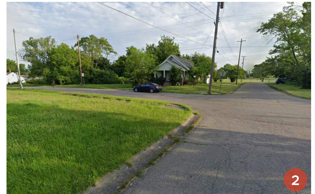
Figure 29 | Residential street lacking marked crosswalks, illustrating gaps in neighborhood-level crossing infrastructure | Google Earth 2025
