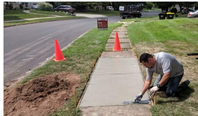
Figure 92 | GSI Concrete, easy and cheap repair to restore neighborhood confidence | Unnamed photographer
